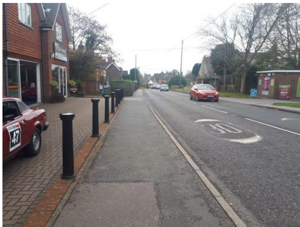
Photograph 3: Footway on the Eastern Edge of High Street
