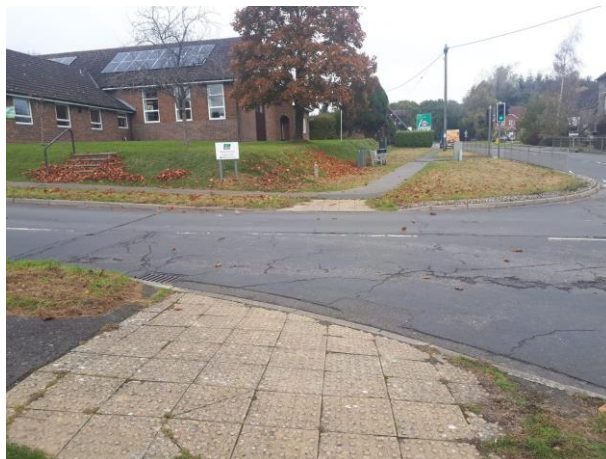
Photograph 1: Oakwood Park Crossing with Dropped Kerbs and Tactile Paving
