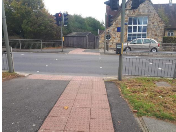
Photograph 2: High Street Pelican Crossing
